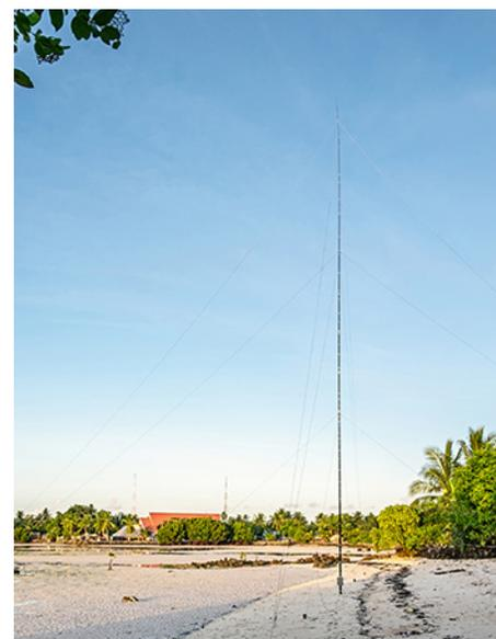
*The 18-meter-high RA6LBS vertical for 160M/80M/60M/40M/30M.*
