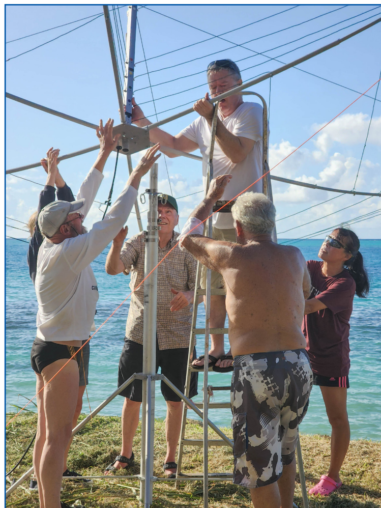
Working together to get the hex beam assembled. Photo: N7BX
